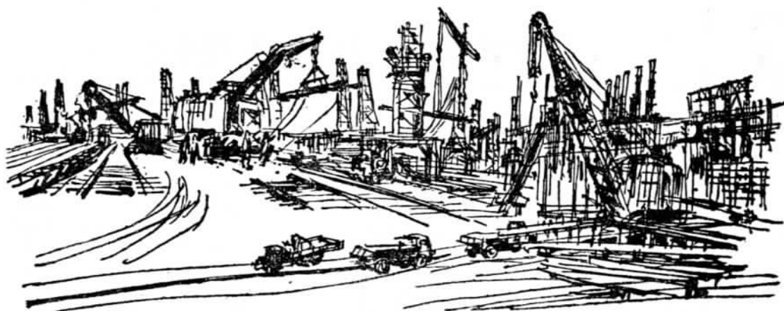
On the Construction Site
