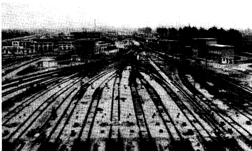
The Jiangcun railroad yard with 75 km of rail, 136 switches and 51 overpasses and culverts services the Hengyang-Guangzhou double-tracked line. It was completed in June 1988.
