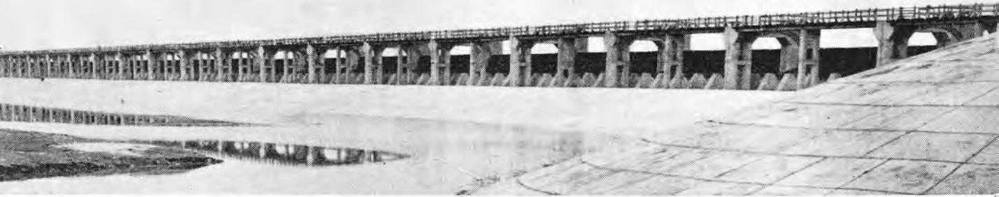
This 1,054 metres long movable dam at Taipingkou with 54 sluice gates controls the flow of water into the Yangtse flood detention basin—it is the biggest dam in China
