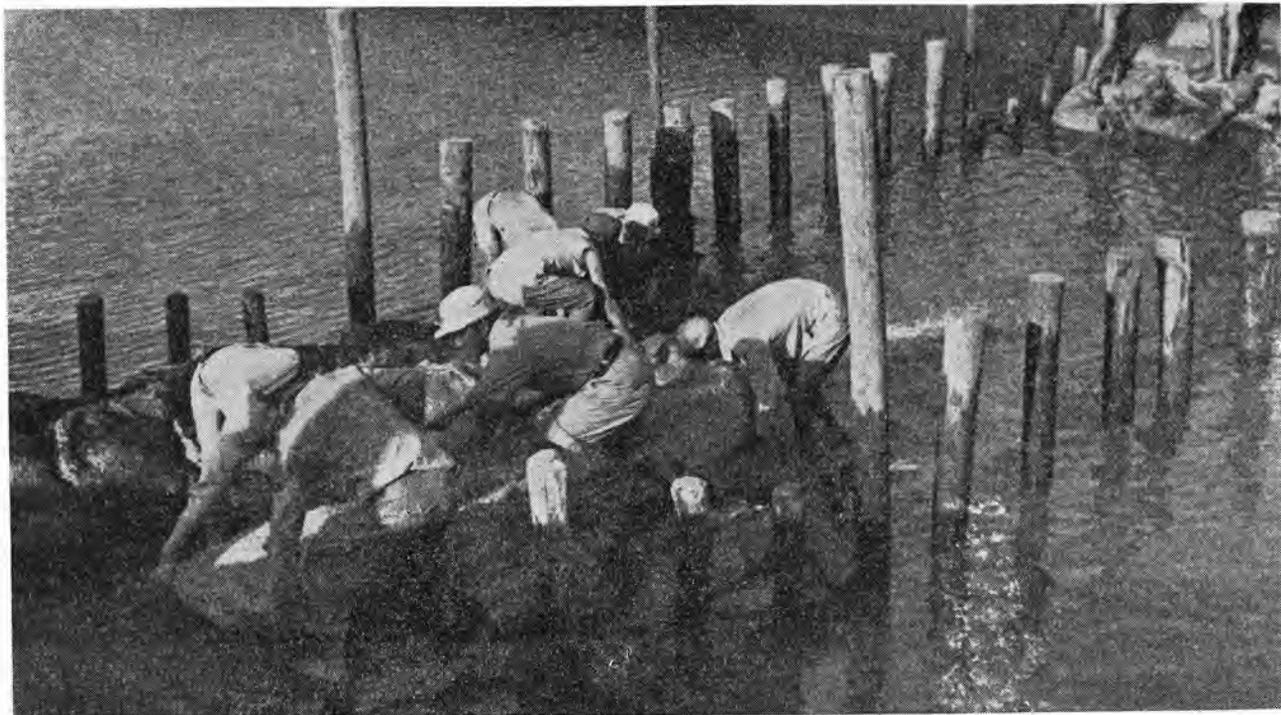
A canal is dammed with sandbags, the first step in building a new irrigation system
