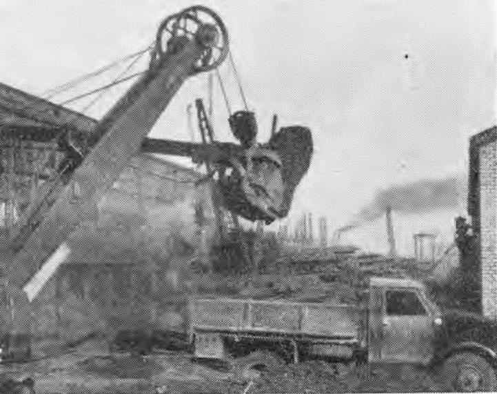
Foundation of new plants entailed moving 100,000 cubic metres of earth. Such work is being increasingly mechanised
